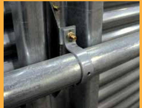
Stiffener connection to sidewall
