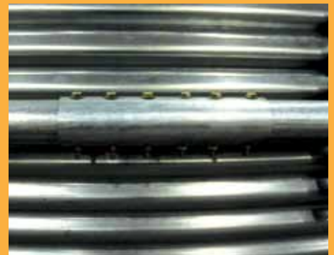
One piece bolted coupler
