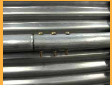
Swaged-bolted splice
